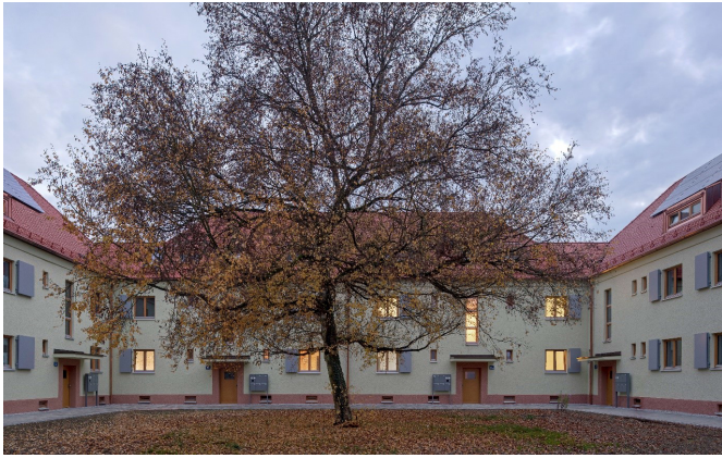
Figure 1. The U-shaped building for the MAGGIE research project after the refurbishment [3].
